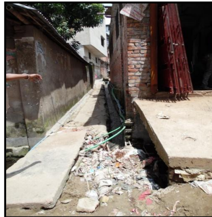
Figure 2.31: Co existence of drainage and water pipelines, Motijhorna hill, Motijhorna. Source: Field survey, August, 2014
