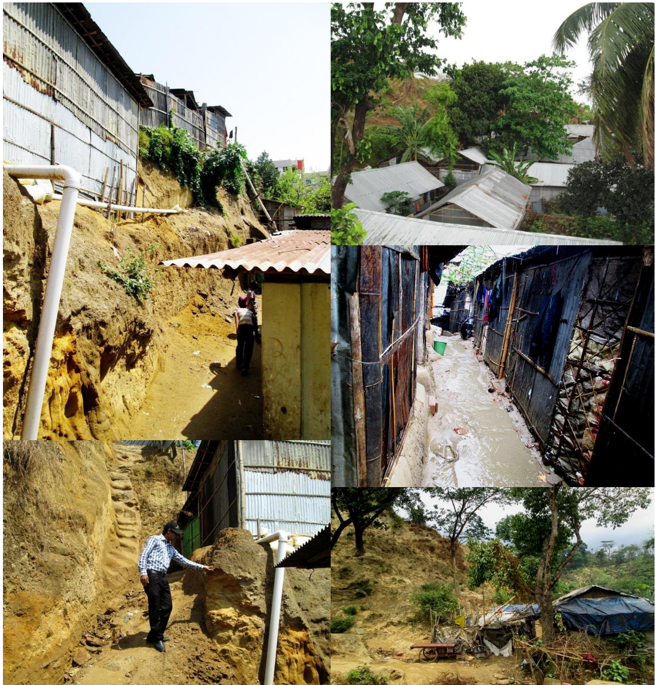
Figure 1.2. Some landslide vulnerable areas of Chittagong City
