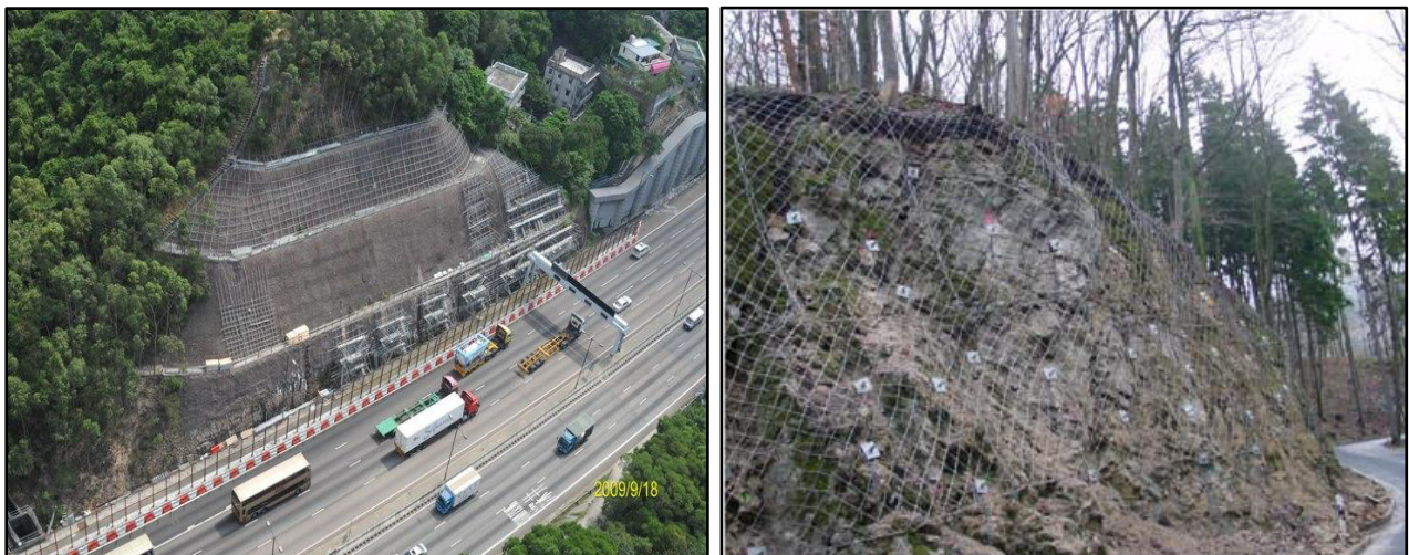
Figure 5.4. Roadside Slope Stabilization by wire mesh (Source: ROTEC Intl, USA)
