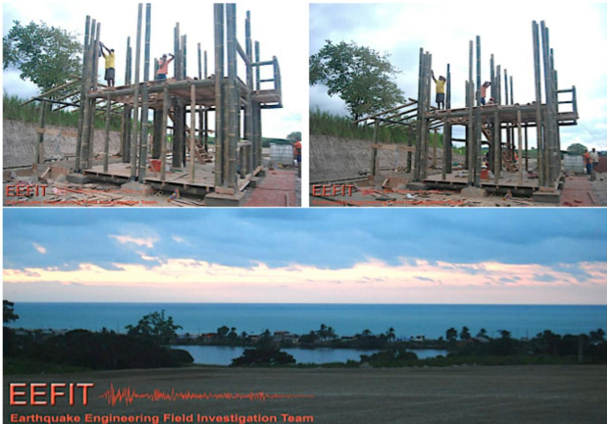
Figure 8-3. Rebuilding a fishing village using bamboo and wood structures. Source: Bayes Ahmed, fieldwork, June 2016
