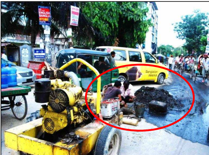
Photograph 15: Road Maintenance in Day Time
