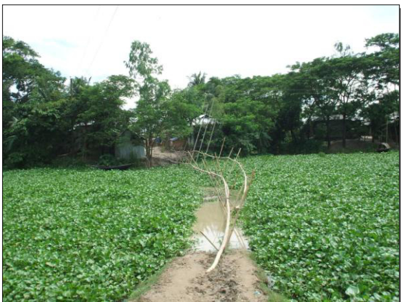
Photograph 05: Poor road way condition
