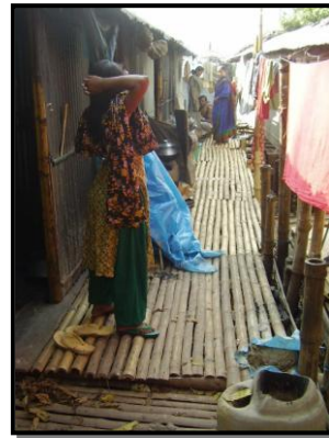
Photograph 4.3: Road made with bamboo
