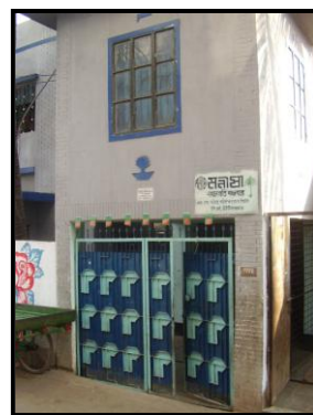
Photograph 4.22: Manisha health center
