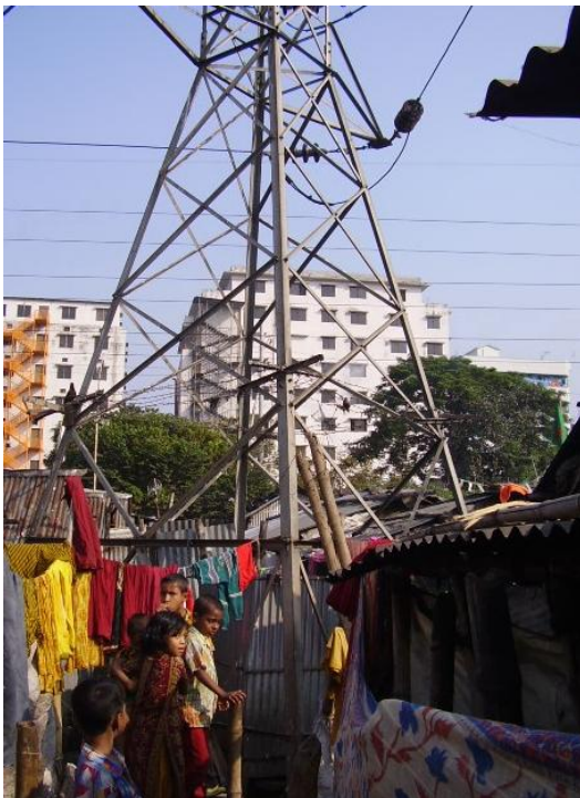
Risky electricity poles
