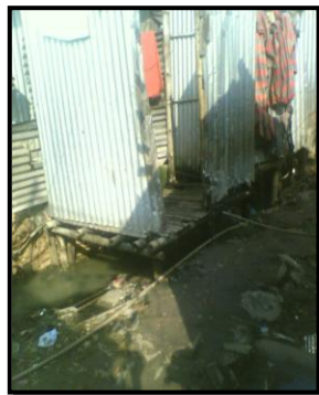
Photograph 4.15: Poor bathing facility
