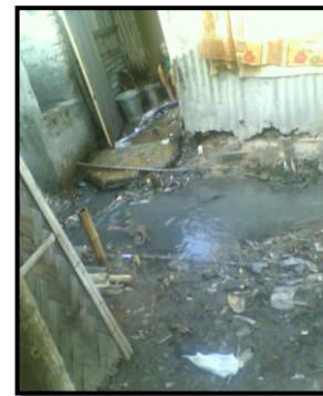
Photograph 4.16: Poor washing facility
